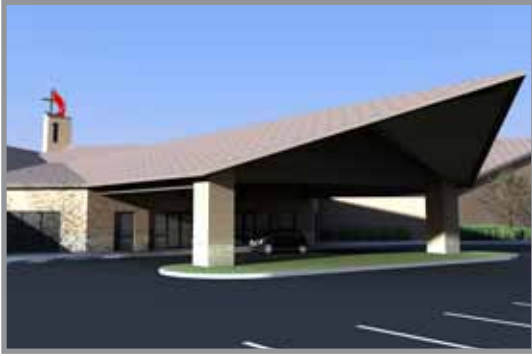
HiFive's work on Mason United Methodist Church includes a new entrance.
